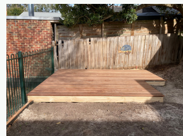
The decking gets laid
